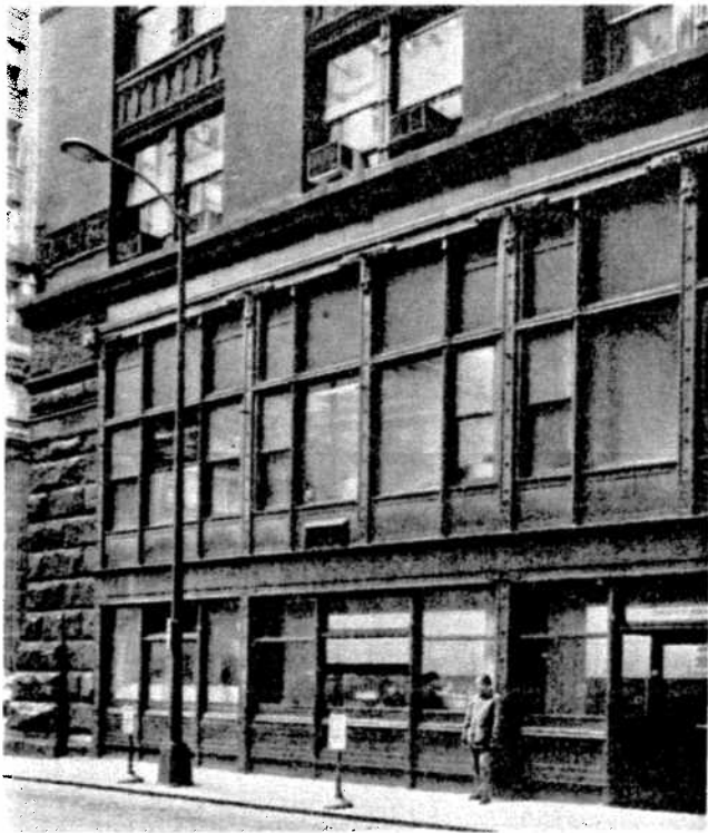
Ribbon windows and skeletal construction of the first two stories along Quincy Street. Note the continuous expanse of glass compared with the limited glass area in the masonry wall above. (Richard Nickel, photographer)
